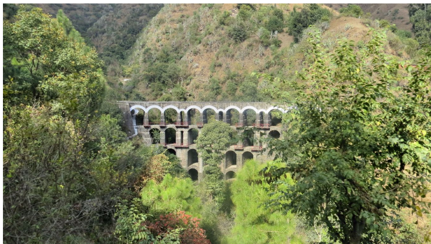
Bridge No 541 near Kanoh
